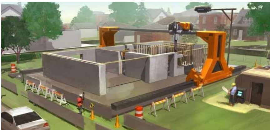
Figure 1: Contour crafting in construction.
