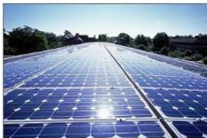
Fig 1.3 A large silicon solar array installed on the roof of a commercial building.
