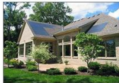
Fig 1.4 Thin-film solar tiles on the roof of a building.
